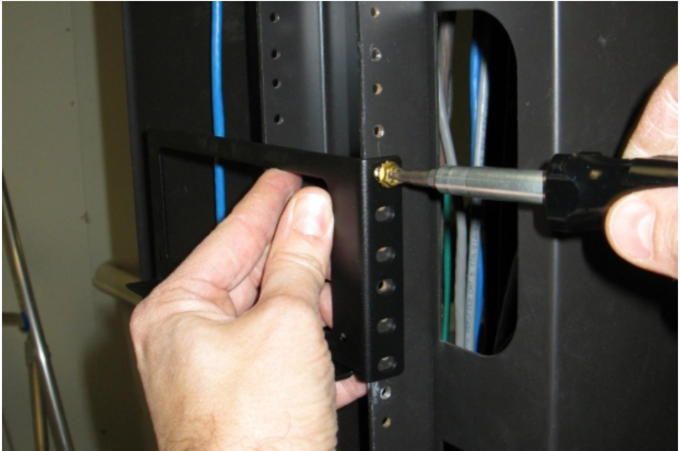
Figure 4.10: CX II/CXi II Controller Rack-Mount Installation - Attaching Brackets to Rack Frame
